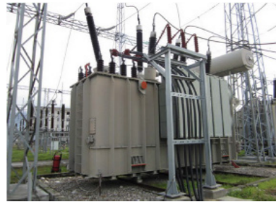
66kV Transformer
