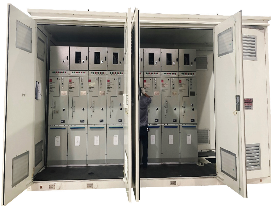
Switchgear inside a secondary substation kiosk
