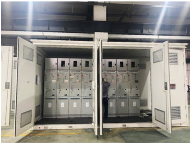
Secondary collector station (MV substation kiosk)
