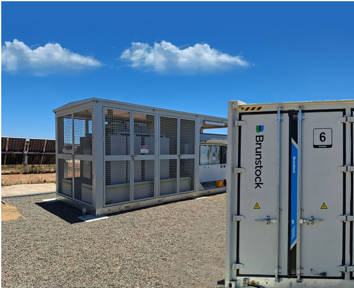
A Brunstock step-up skid station and battery energy storage system delivered in 2025 to a site in South Australia
