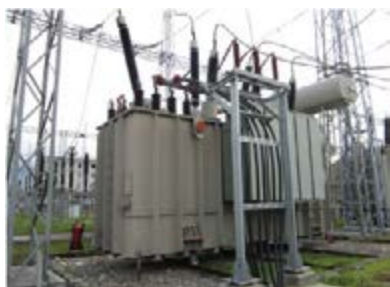
66 kV transformer
